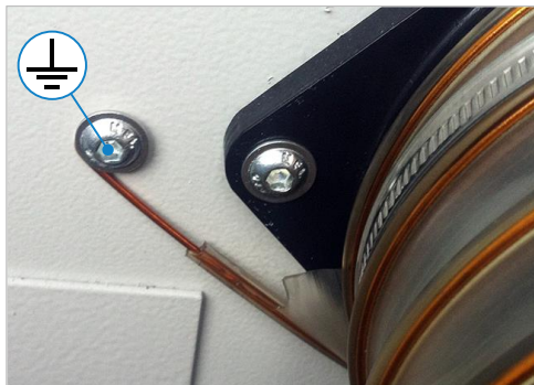
Figure 19: earthing example for suction hose
